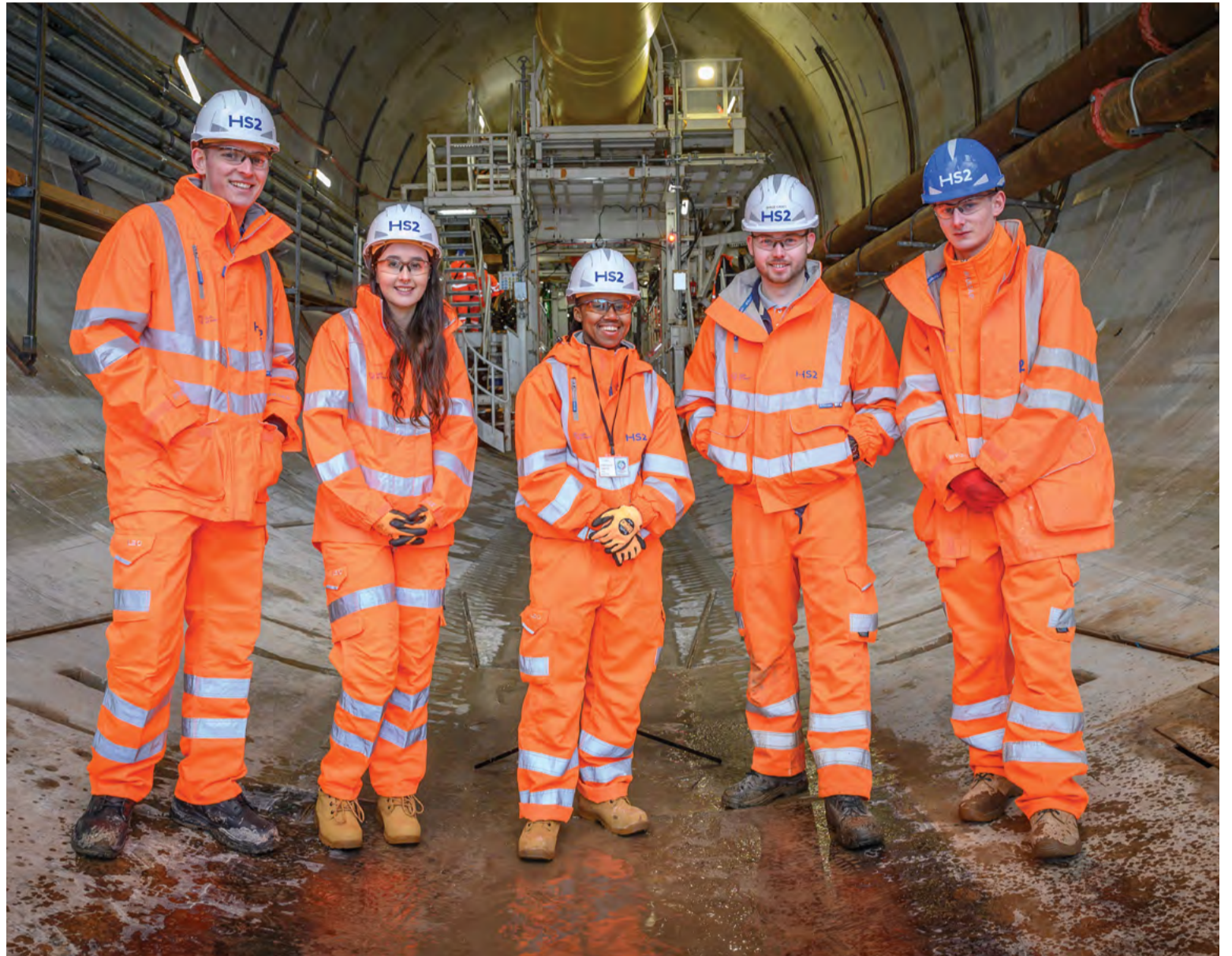
Apprentices pictured inside the tunnel portal at HS2's Long Itchington Wood site. (Image: hs2.org.uk)
