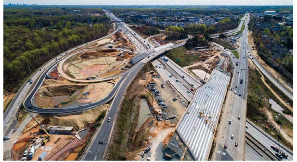
Ongoing construction at the Route 50 interchange with Interstate 66 in Fairfax, Virginia, US. (Image: EPA-EFE/Jim Lo Scalzo)
