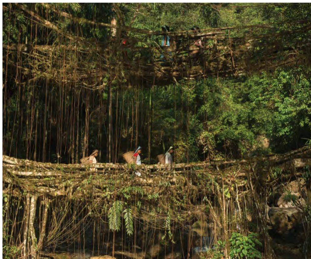
Rubber trees in Meghalaya, India, are trained by the Khasis to grow into bridges across rivers that swell during monsoons. Visually stunning, the bridges are a symbol of how humans work with, not against, nature.
