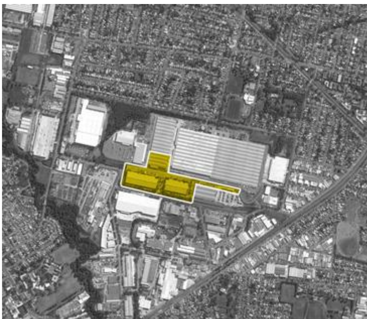
Figure 4.7 Yennora Intermodal Terminal
