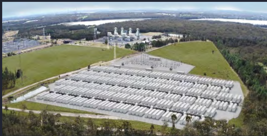
The new Waratah Super Battery will be capable of discharging up to 850MW/1680 MWh. (Image: Powin)
