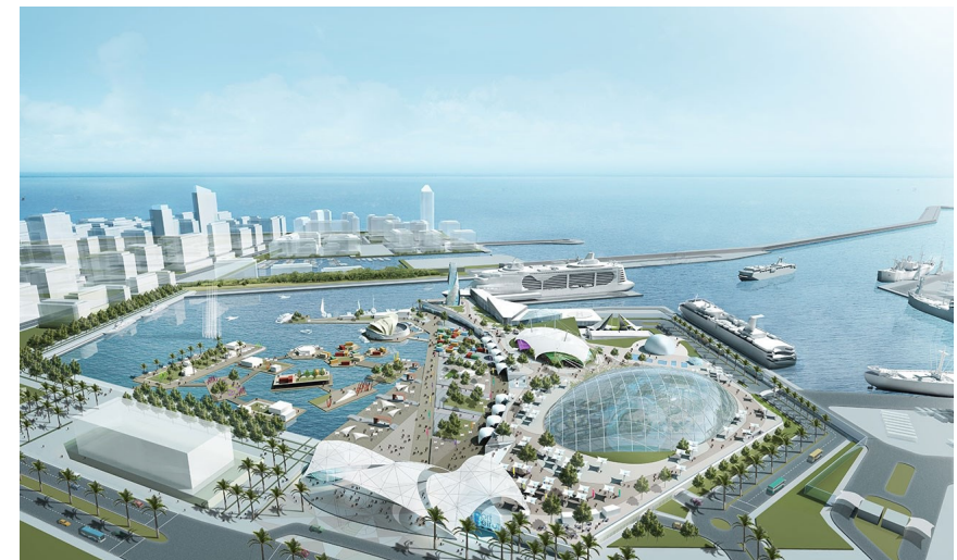
Port of Beirut rehabilitation and extension. (Image: dar.com)
