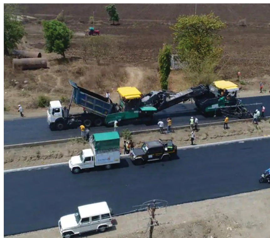
A section of the new road in Maharashtra. (Image: Twitter)
