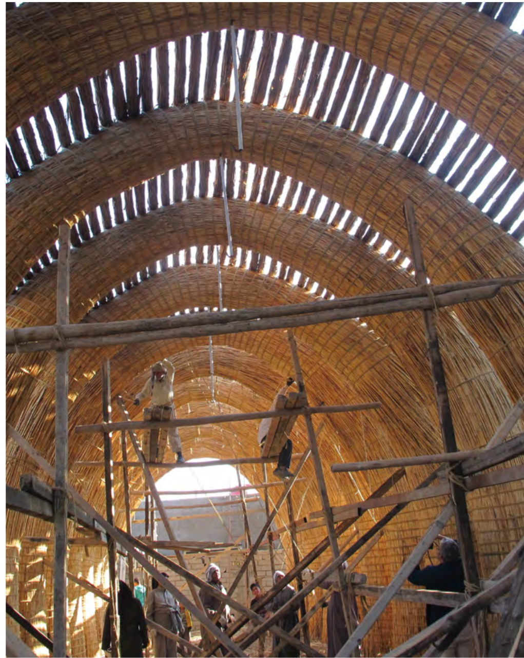
A Ma'dan house (mudhif) in the southern wetlands of Iraq, built of qasab reed without using mortar or nails, can be taken down and re-erected in a day.
