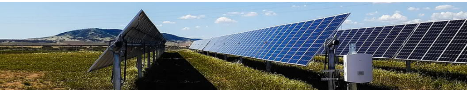
South Hummocks SA, Solar Farm – 5 MW grid connected solar farm project. Source: MPower
