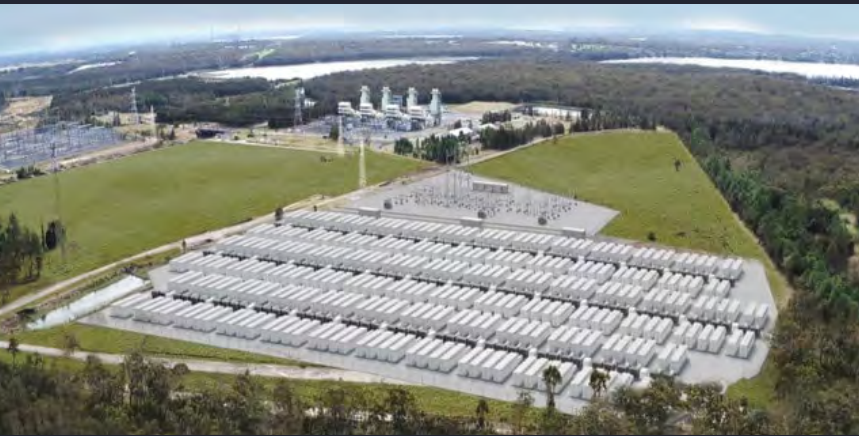
The new Waratah Super Battery will be capable of discharging up to 850MW/1680 MWh. (Image: Powin)
