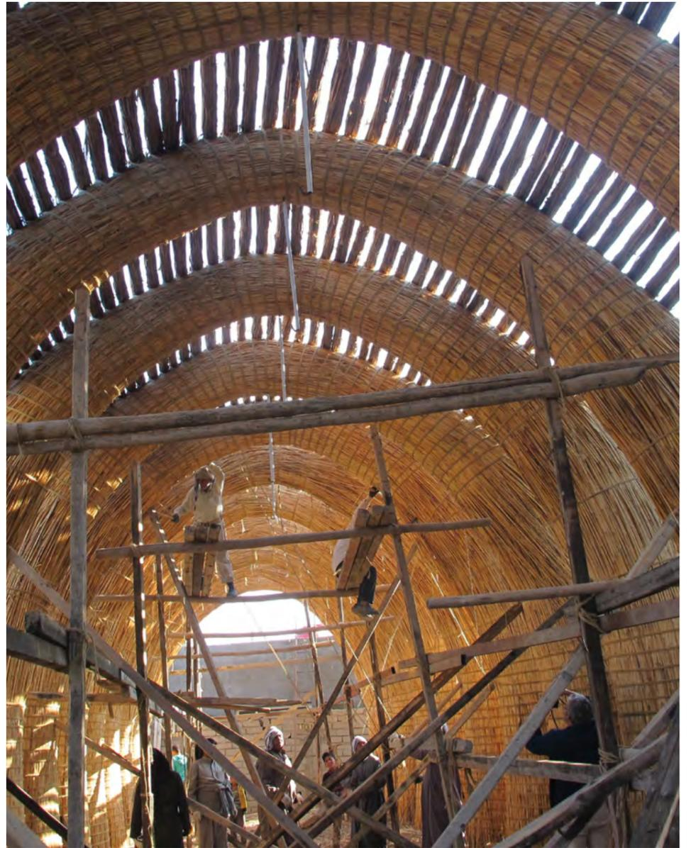
A Ma’dan house (mudhif) in the southern wetlands of Iraq, built of qasab reed without using mortar or nails, can be taken down and re-erected in a day.
