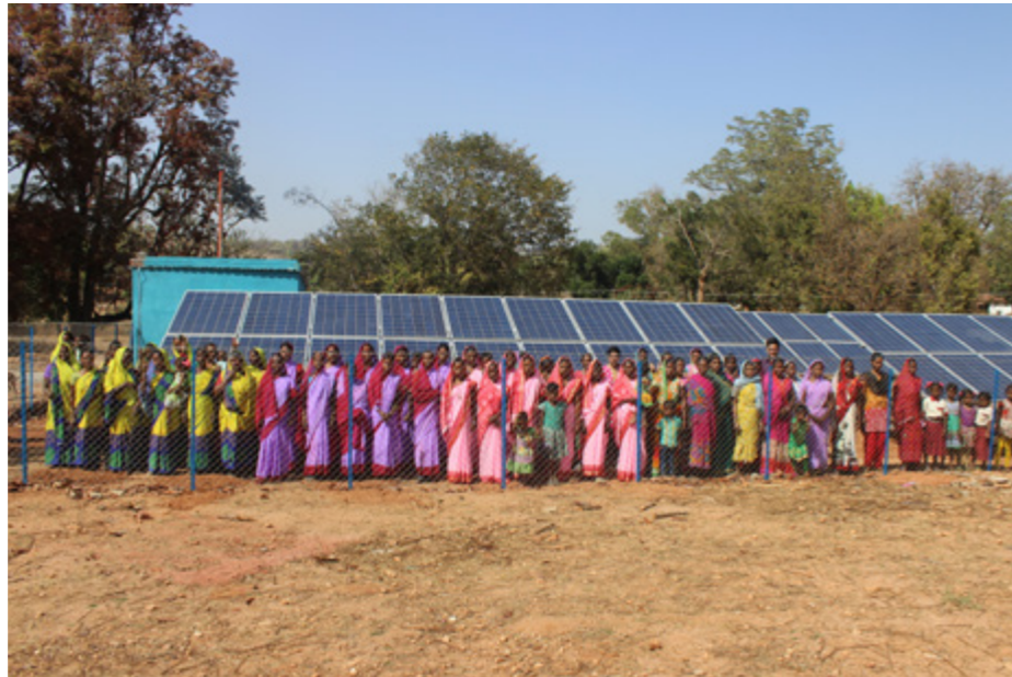
Photo courtesy : Bank of America
