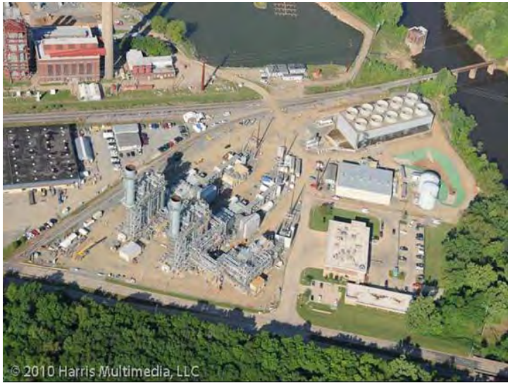
J. Lamar Stall Combined-Cycle Gas Plant
