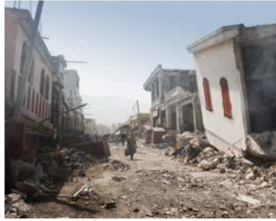
Partners In Health Haiti 2010 Earthquake
